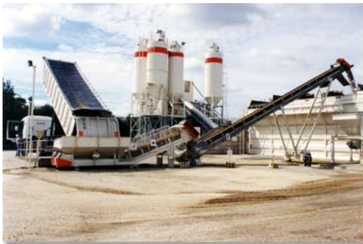
Illustration 1: Centrale à béton - photo UNICEM
